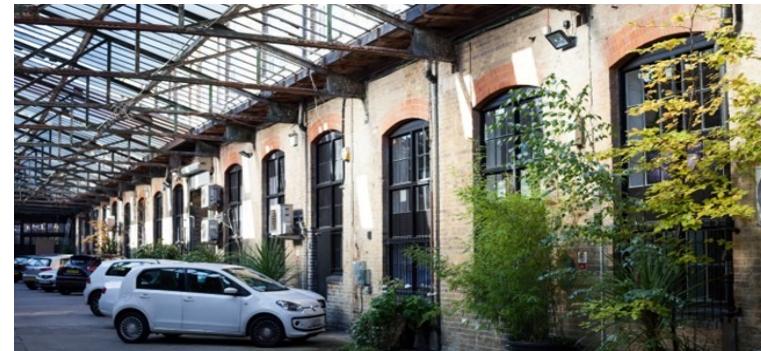
Busworks - United House
